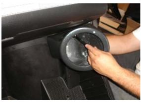
Once the holes are drilled, mount the kick panel using the supplied hardware
